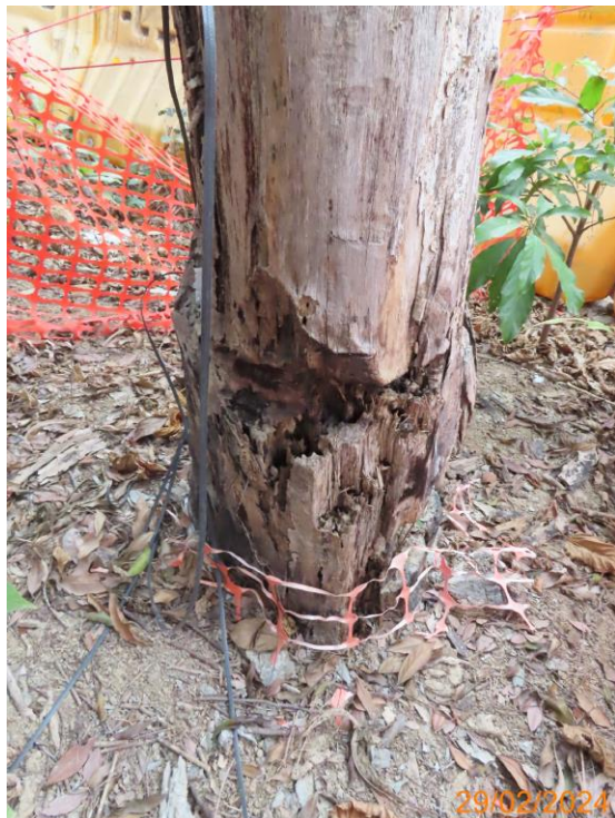
11: U041_Wood damage by termite
